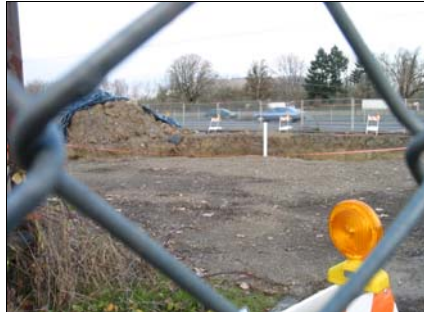
Site of Future SeSequential Biofuels Renewable Fuel Pump Station.
